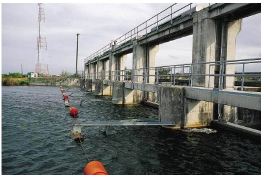
FOUR WATER-CONTROL GATES, including this one, punctuate the Tamiami Trail, which runs across southern Florida from east to west. The gates regulate the amount of water that flows south into Everglades National Park.
